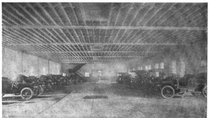
INTERIOR OF THE GARAGE OF THE AUBURN AUTOMOBILE CO.
